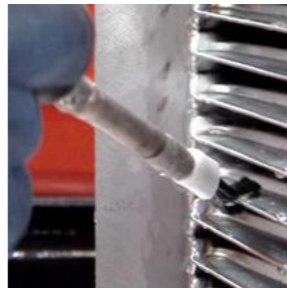
Cleaning of areas which are hard to reach
